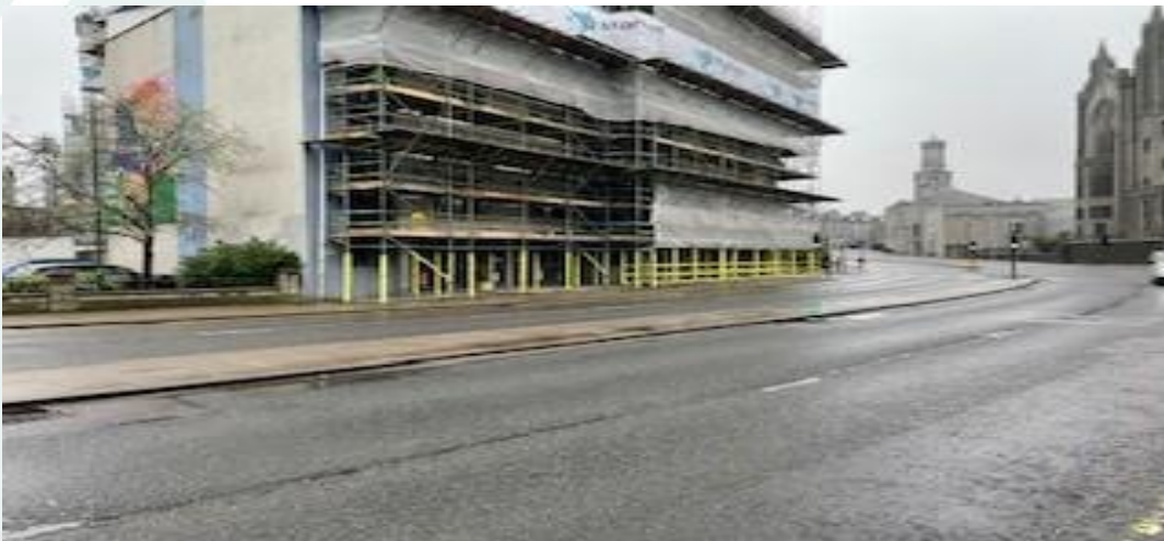
lane closure and footpath restrictions now removed.
